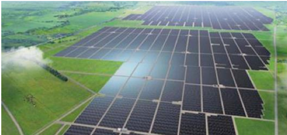
Figure 3 - Nzema Solar Plant (image from pv-magazine.com)
